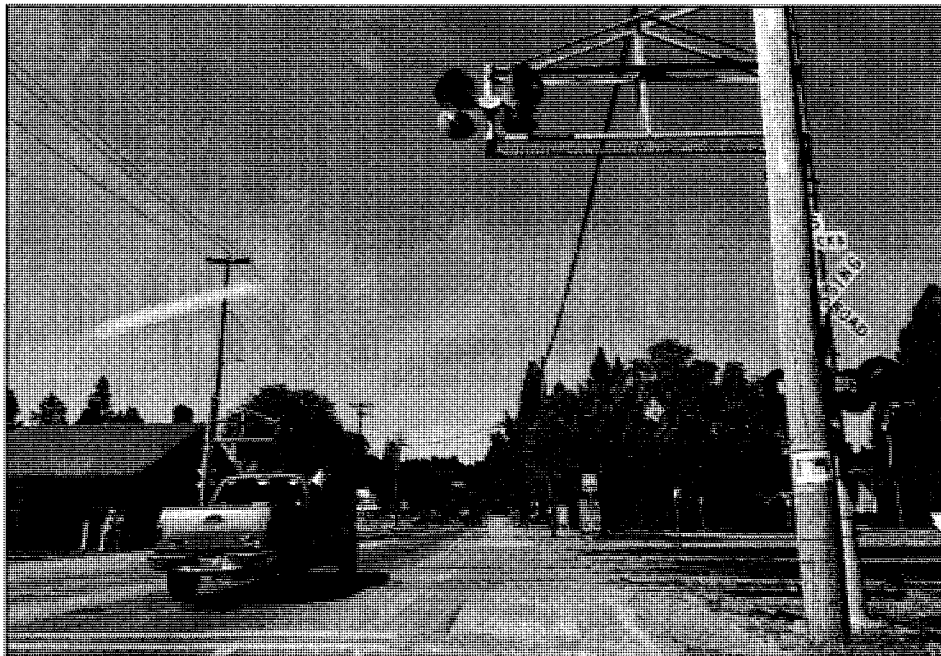
View at mile marker 139.5 facing west along Commercial Street
