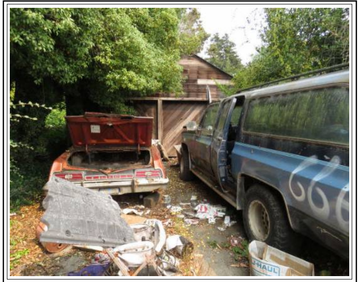
Detached garage structure located on the subject site.
