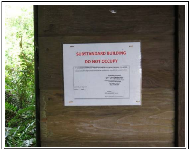
"Red tag" on subject residence.
